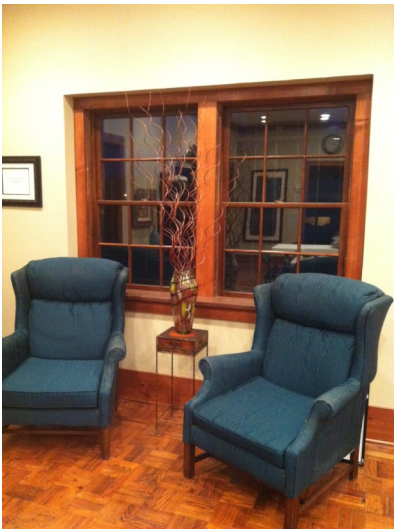
[Left] The office also highlights the new energy-efficient wood windows crafted by Wewoka Window Works. Donated and installed by Dennis Myers, the windows replicate the originals in place throughout the three rooms. In addition to the windows, low-voltage lighting and new blown attic insulation have dramatically increased our energy efficiency.
